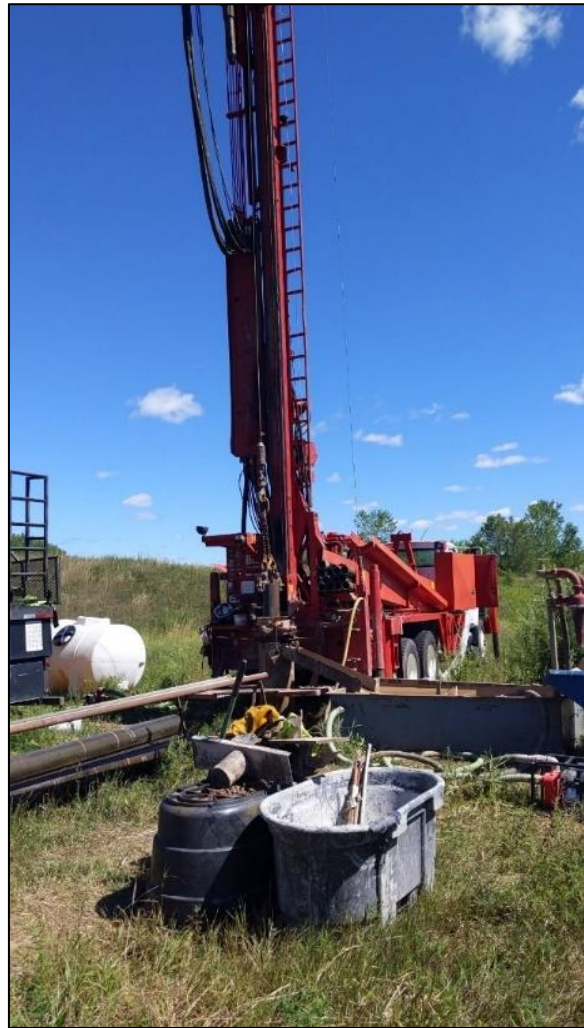
Mud Rotary Rig Installing SC-6
