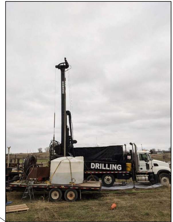
Sonic drill rig set up at G-6
