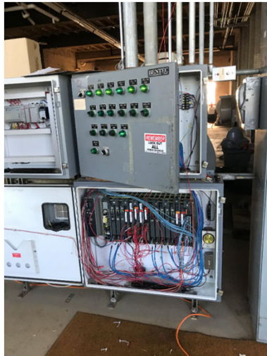
Decommissioning of Control Infrastructure
