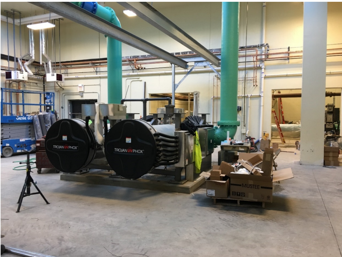
Photo 4. The new Trojan UV PHOX system at the New Brighton Treatment Plant.
