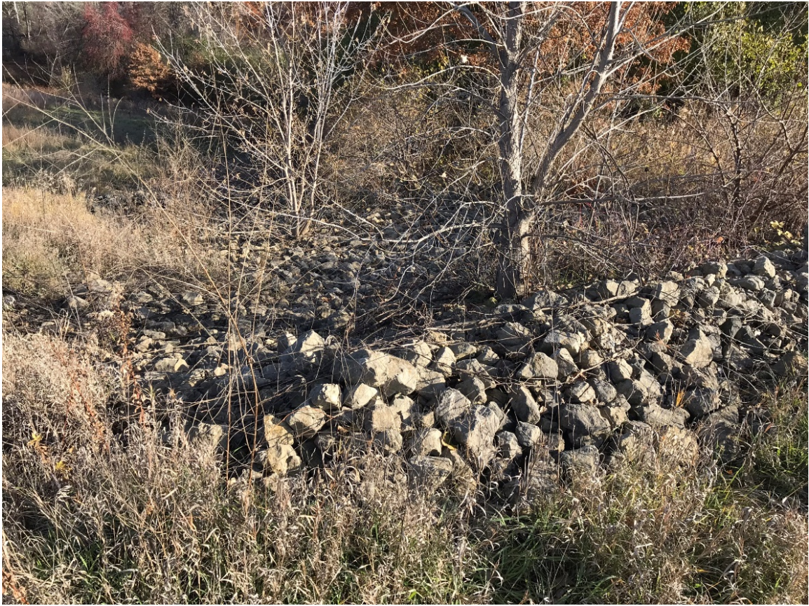
Photo 41. Rip rap for mitigation of run-off from an upper road at Site 129-15.
