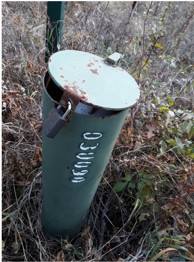
Photo 27. Well 03U090 at Site F shown with a broken lid.
