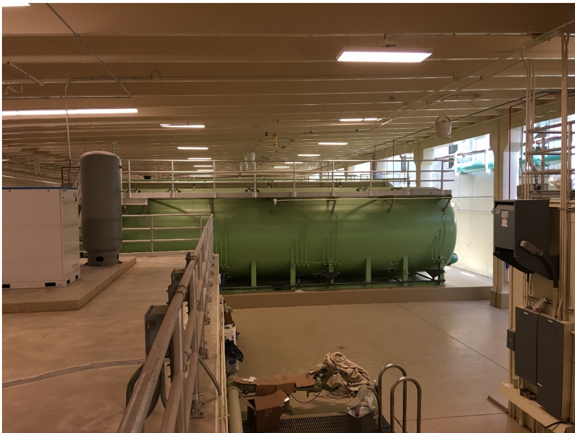
Photo 2. Part of the New Brighton iron and manganese pressure filtration system.
