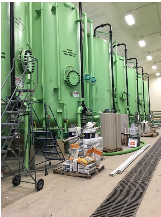
Photo 5. Granulated Activated Carbon (GAC) tanks at New Brighton Water Treatment Plant.
