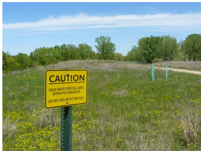
Signs, like the one in the photograph, mark areas where land use controls are required as part of the remedy to help ensure protection of human health and the environment. A groundwater monitoring well, surrounded by protective posts, can also be seen in the photograph.
